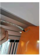
6. Remove the plug from the power supply. Labeled wire is Minus.
